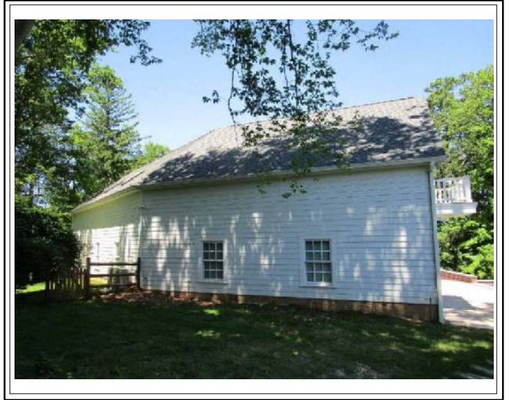
5/Car Detached Garage - Rear Photo #2
