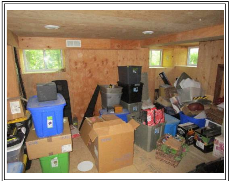
Basement - Unfinished Area - Photo #2
