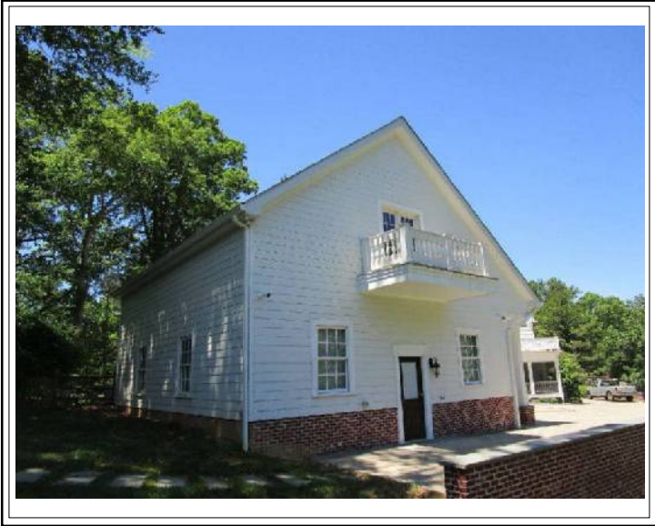
5/Car Detached Garage - Rear Photo #1
