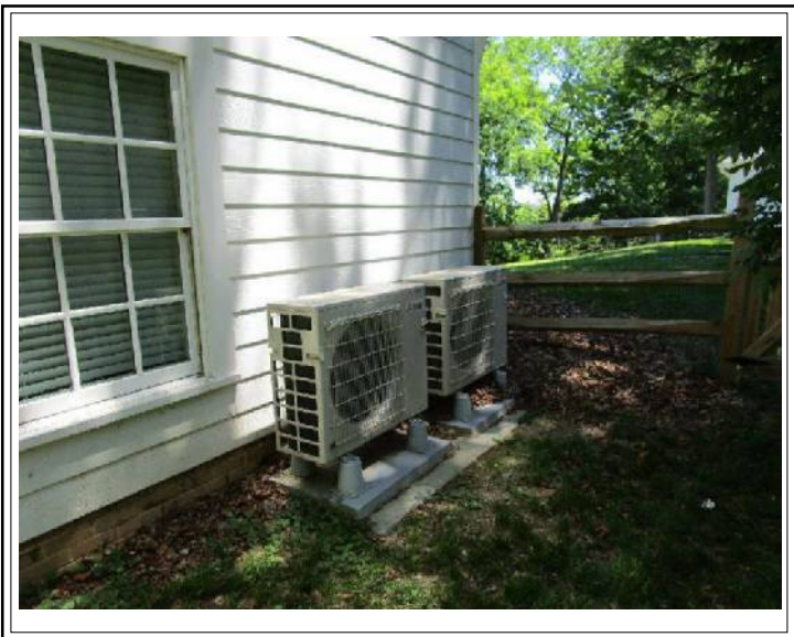
5/Car Detached Garage - Condensers
